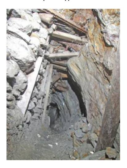
Slightly further is a point where we thought that we were breaking through, we were in fact correct but it was only about 10 feet of clear passage. Then another fall. This point had several faults coming together and the collapses here had formed a chamber. The big problem was relocating the adit, a matter of guesswork. We drove through the collapsed chamber timbering our way forward.
