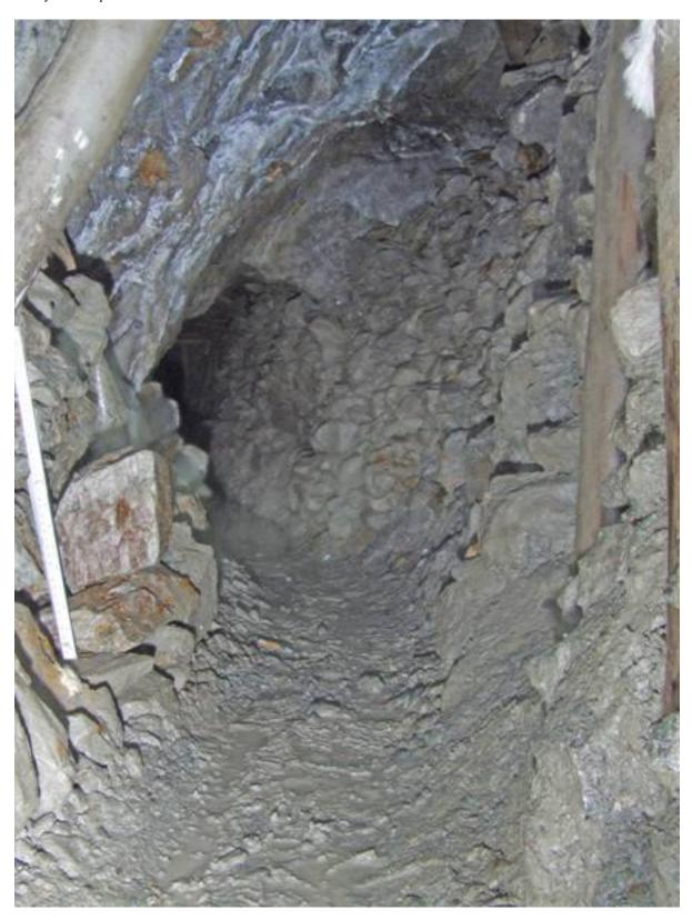
And below, 'the crack' with its urethane grouting. A good place to get out of.
