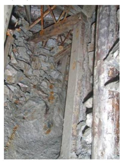
At the very back just to the left of the rock is the backfilled forhead, our roadway turning right in an attempt to re locate the continuation of the adit west.
