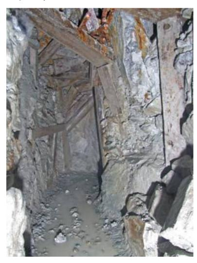
Concrete a plenty here, as it crossed yet another fault. Right and left is all concrete. At this point the roadway turns back to the right and picks up on the fault that the adit most certainly followed.
