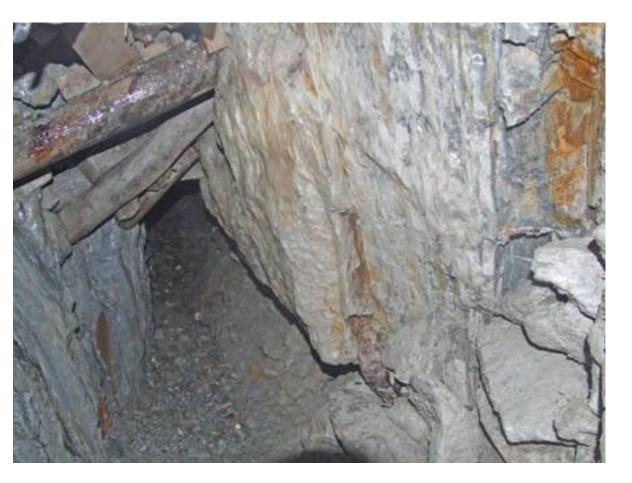
This is on the fault itself. Footwall on the left, hanging on the right. The cleavage and bedding plane are on the same plane here, on the left it about 60 degrees to that on the right.
