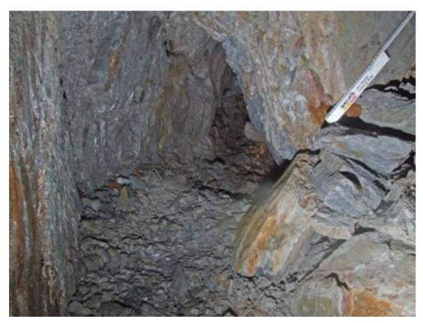
Below is the end of the road. You will have to look carefully to make anything out. On the floor are pieces of rotten timber. On the right is a huge slab that has come crashing down. If you look very carefully you will see pieces of rotten timber trapped between the slab and the roof. Look high centre right.
