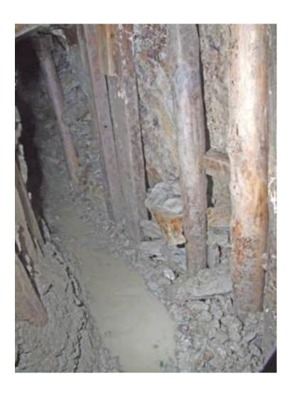
Just past this point there is a large crack in the hanging wall, the timber on the right is helping to support this, behind the timber the crack was urethane grouted.
