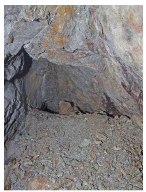
Eventually we reach the drystone arched section. Here there must have been some bad ground, or possibly old mans workings. In places along the adit a barren vein or fault can be seen, it's possible that this may have been worked near to the portal.
