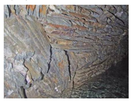
See how the arching has been built into the rock on the left
